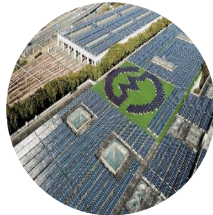
Longyang road metro station PV project, Shanghai, 3.66MW
