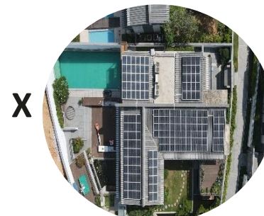
Family green power PV & ESS project, Dongguan, 30kW
