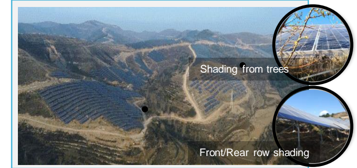
Project: XX PV plant in a coal mining subsidence area of Yangquan, Shanxi
